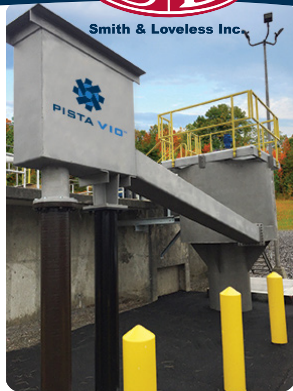
The PISTA VIO™ is available with stainless steel tankage or with traditional concrete. Models handle flows from 0.5 to 100 MGD.
