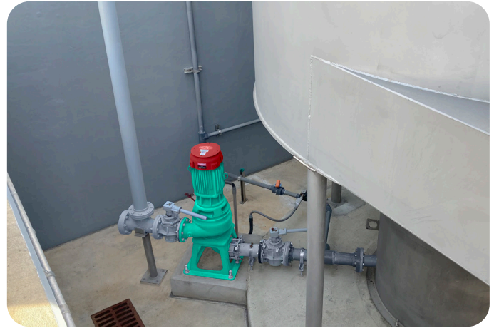
The PISTA® TURBO™ Grit Pump shown above in its remote-mounted configuration is the industry's only true pump designed exclusively for wastewater grit handling.
