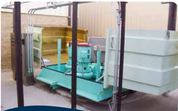
EVERLAST™ TRIPLEX 3-Pump Station to Help Meet Special Flow Conditions
