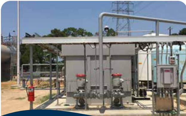
STAR ONE™ Non-Clog Pumps Heavy-Duty Solids Pumping Placed Above the Wet Well
