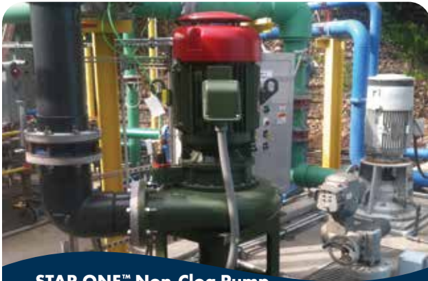
STAR ONE™ Non-Clog Pump Heavy-Duty Solids Pumping Placed Above the Wet Well
