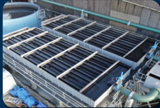
Lamella Clarifier – Steel Manufacturing Queensland
