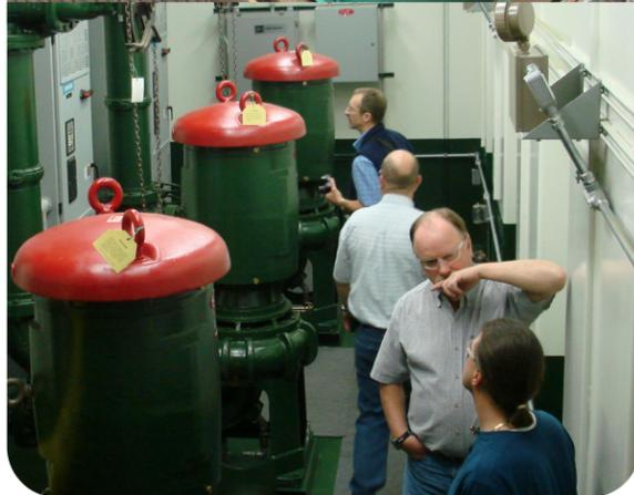
The **CAPSULAR**® Underground Pump Station provides an operator-friendly and economical solution for large-flow pumping (with multiple S&L Non-Clog Pumps) up to 20,000 GPM / 1,262 lps when compared with more expensive concrete, built-in-place stations. With exclusive Safe-Stair entryway module and integrated HVAC, the pump station design meets the OSHA definition of “designed for continuous human occupancy” and therefore does not require classification as *confined space entry*.
