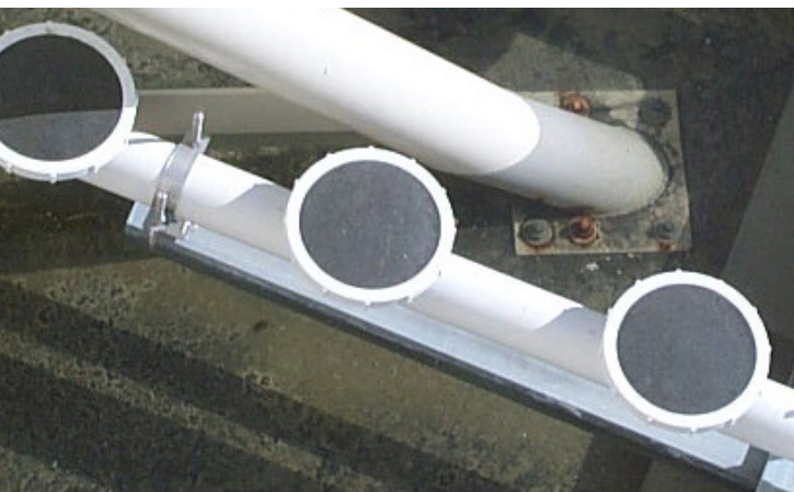
Close-up view of a circular fine bubble diffuser recently installed on a S&L retrofit project.
