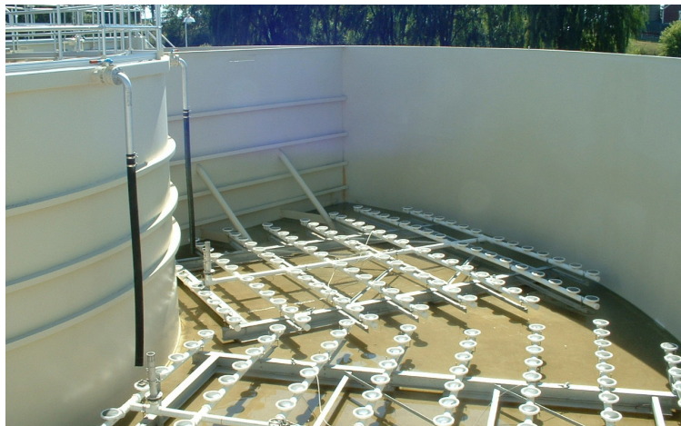
Replacement circular fine bubble diffusers were installed during this S&L retrofit project.
