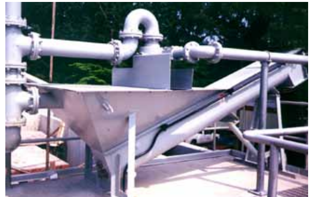
The PISTA ® Grit Screw Conveyor (shown above and below with a PISTA ® Grit Concentrator) effectively washes and dewateres grit for disposal —all with hassle-free operation.
