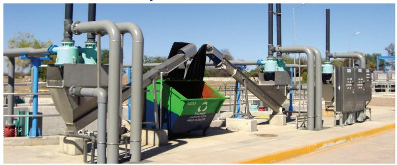
The **PISTA®** Grit Screw Conveyor is designed to work in concert with the complete **PISTA®** Grit Removal System, providing superb dewatering &
