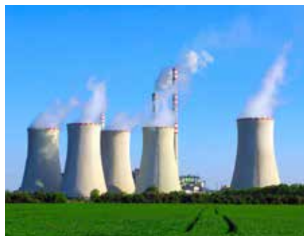
At this coal and natural gas power plant in the United States, S&L provided two Model 12 PISTA® Grit Chambers to remove rocks and sand from river intake.
