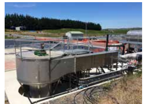
S&L can provide both concrete or steel grit chambers for implementation in any industrial intake system like this one in Australia.
