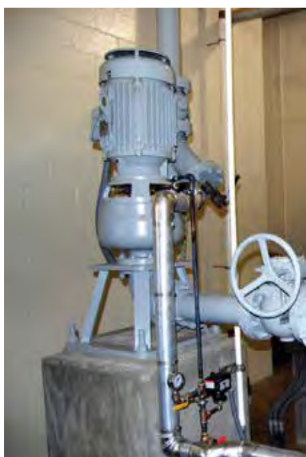
Remote-mounted, Flooded Suction Turbo Grit Pump
