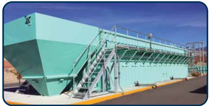
Above, Factory-built and then shipped complete to the project site. Below, models can be arranged for containerized shipping.
